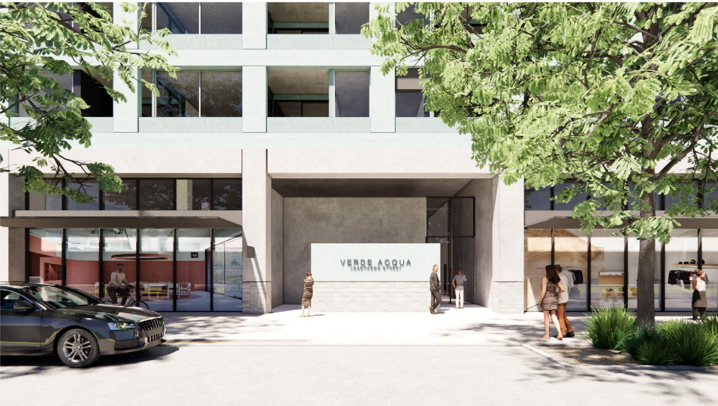
BUILDING A ENTRY
