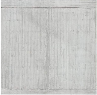
CO-4 OFF-FORM PRECAST CONCRETE FINISH
